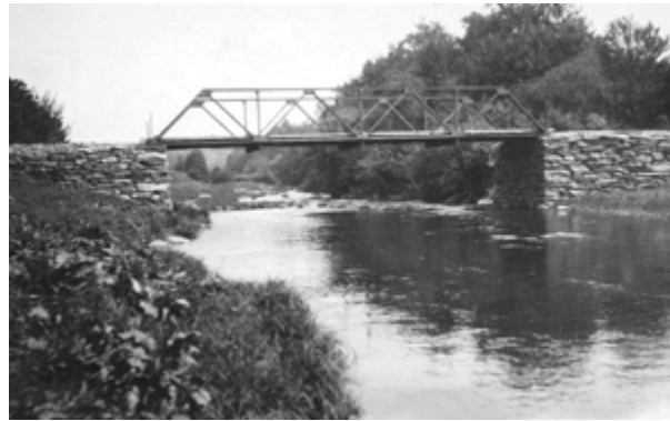
Bridge at Slater Farm, current Farber Farm; from the Alvena Hitchcock Collection.
