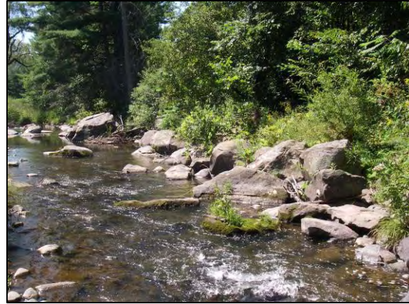
Revetment at Stations 9900-9779
