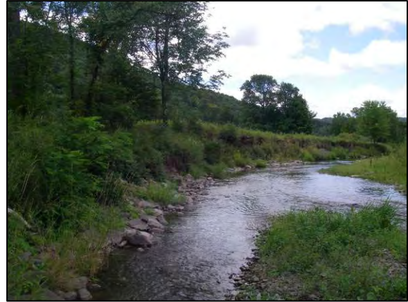
Erosion at Stations 15274 - 14944
