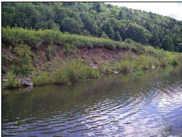
Erosion at Stations 14180 - 14043
