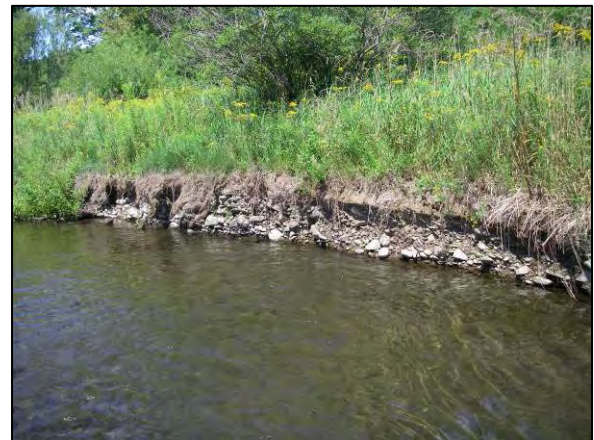
Erosion at approximate Stations 13050-12960
