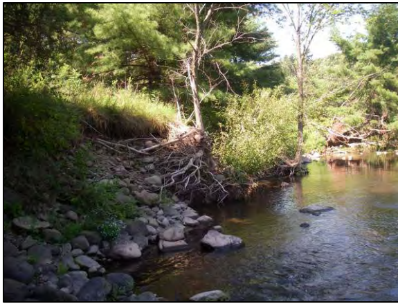
Erosion at Stations 10630-10266
