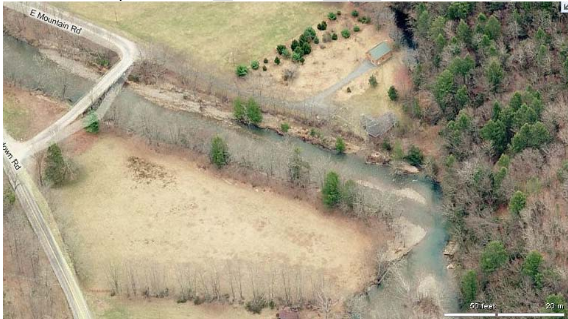
Figure 4 90 degree right turn in stream channel
