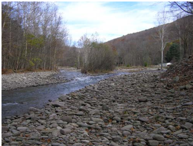
Figure 4 Historic aggradation, channel shifting upstream of Ballace Road Bridge, MU9
