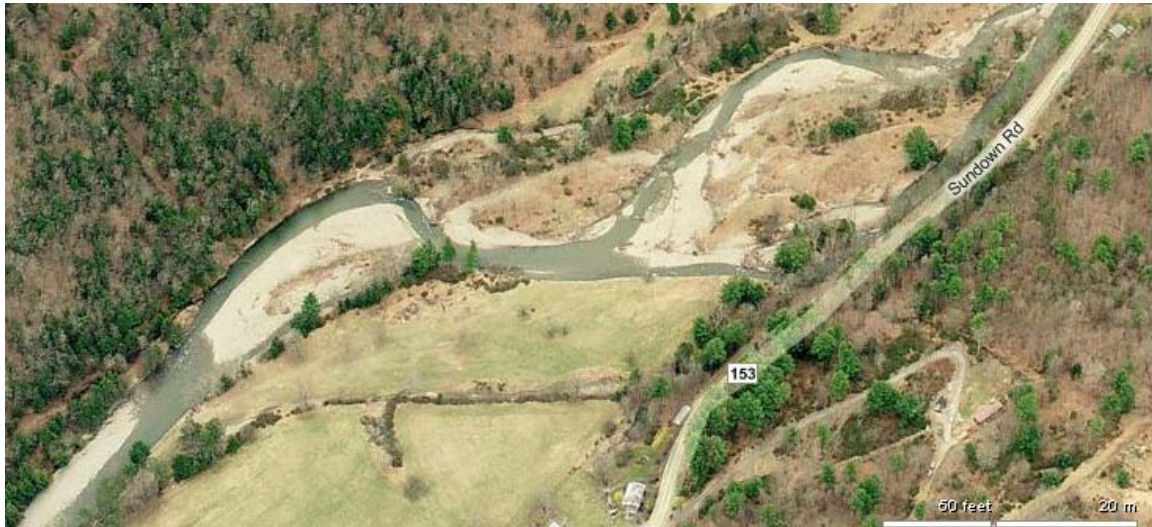
Figure 1 Proposed Rondout Creek Demonstration Restoration Project, looking downstream
