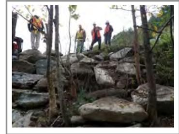
A revetment, purpose built to protect the up stream end of the crib wall, was constructed of large stones, angled back and into the bank to anchor the entire assembly of wood, willows and plantings. More stones were placed at the base along the stream bank for additional protection against scouring during high water events.
