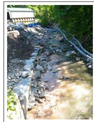
The contract specified for dewatering pumps with a minimum discharge of 20 cubic feet per second (cfs) be maintained to by-pass water around the construction site. Additionally, in an emergency flooding event, the contractor was to supply pumps capable of discharging larger flows of 50 cfs within 24 hours notice.
