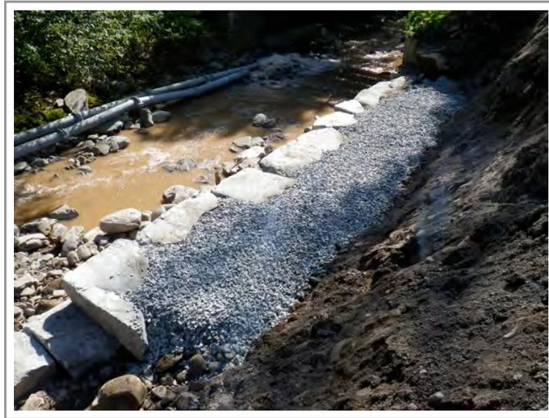
This is the first section of the stone wall that has been brought up to height and is ready for the beginning of the white oak crib wall. It is pitched back one foot for every four foot in height. The wall follows a 2% grade which matched the grade of the stream at this location.
