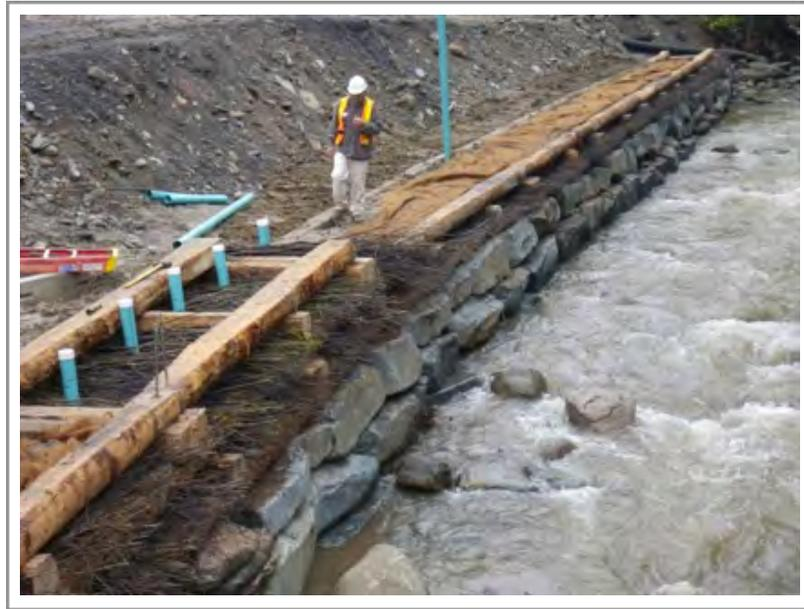
This photo illustrates the various components in the wall. The base stone rising to bankfull height. The crib wall being constructed layer by layer each course composed of willows, soil and fabric. Note the blue watering pipes just in front of the rear oak log. The soil can be observed to fill the entire void behind the crib wall.
