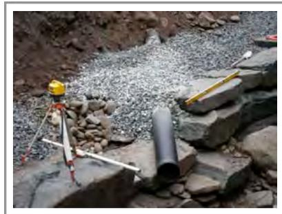
Large quarried stones were shipped to the site to be used in the construction of the base stone wall. The first section of wall with its gravel fill was used to create a base for the installation of the first oak cribbing logs. This ductile iron drain pipe being set connects to the catch basin at the end of the trench drain.
