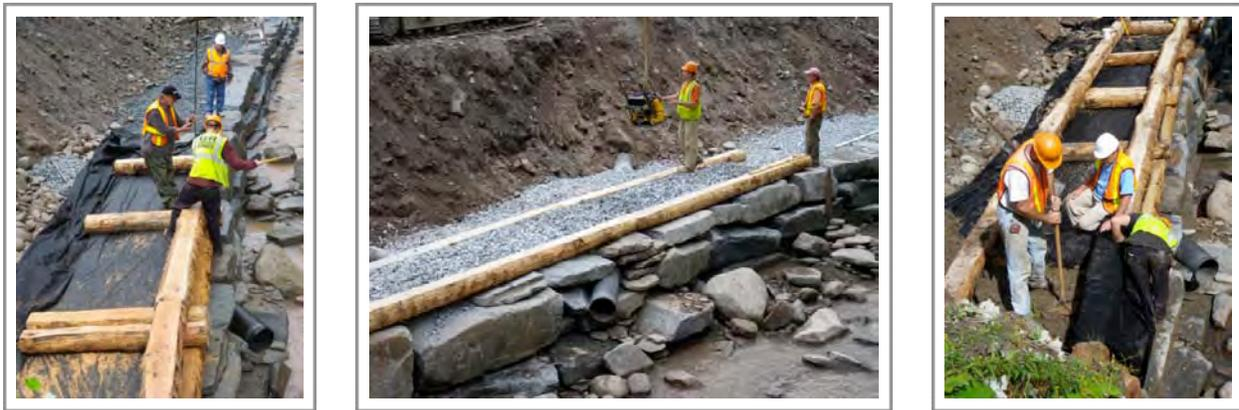
The first white oak logs are set on top of the stone wall. Landscape fabric is applied over the first layer. The logs are drilled and pinned with #6 reinforcing bar. The first layer of soil is being placed and compacted.
