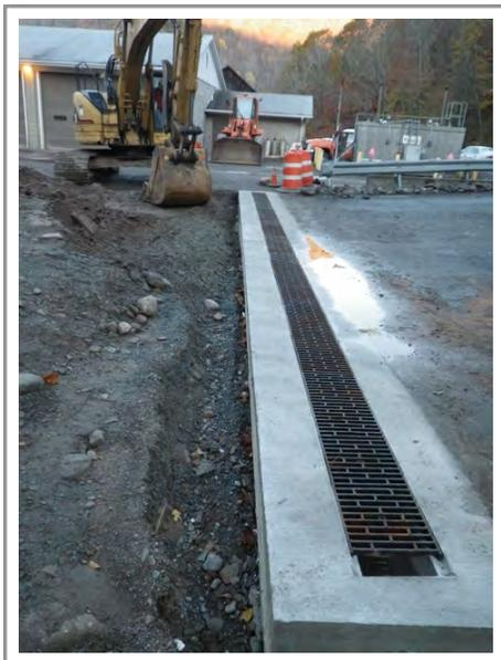
A trench drain was constructed in front of the Ulster County Highway Department salt shed to catch and direct runoff from the salt shed and loading area into the settlement pond which existed on site.
