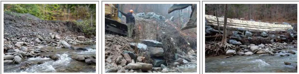
Section C, the largest area to be restored, is embedded with root wads and large stones at its base. Willow clumps are planted among the large stones and root wads. Fascines are planted in the soil area above and native plants intersperse the upper area.
