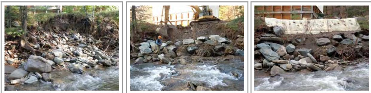
Section B is implanted with several root wads bracketed with large stones which are planted with willow clumps. Willow fascines are planted in horizontal rows above the stones and native plants are planted toward the top of the restored area.
