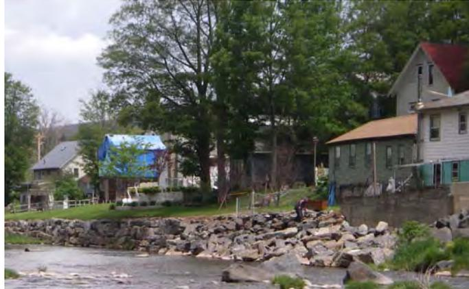
*Streamside development and mowing to the edge of the stream leads to bank failure. This bank has been reinforced with riprap and concrete.*
