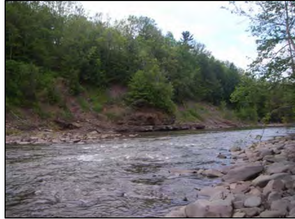
Bank erosion at Station 59100
