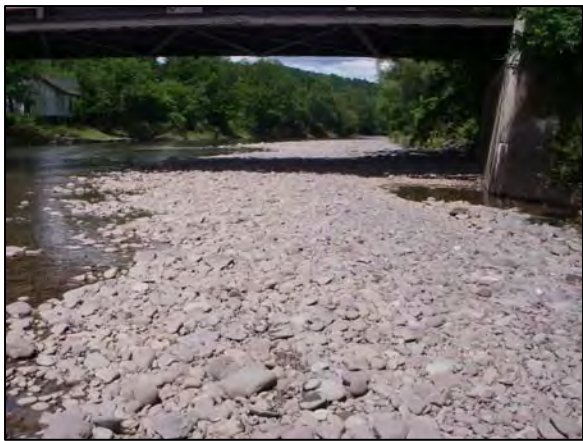
Aggradation at County Route 42 bridge Station 55350
