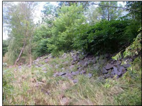
Rip-rap at Station 56600
