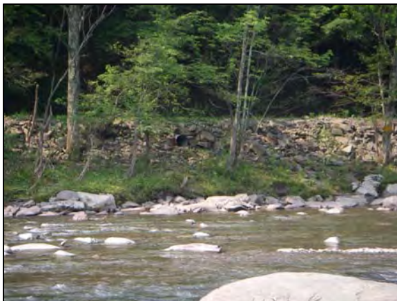
Rip-rap at Station 42050
