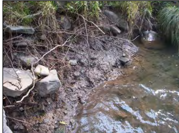
Clay exposure at Station 43800
