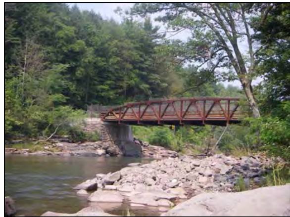
Mosquito Point bridge at Station 41722
