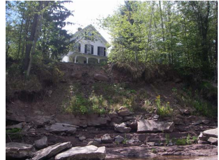
Left Bank, where VRSS would be installed
