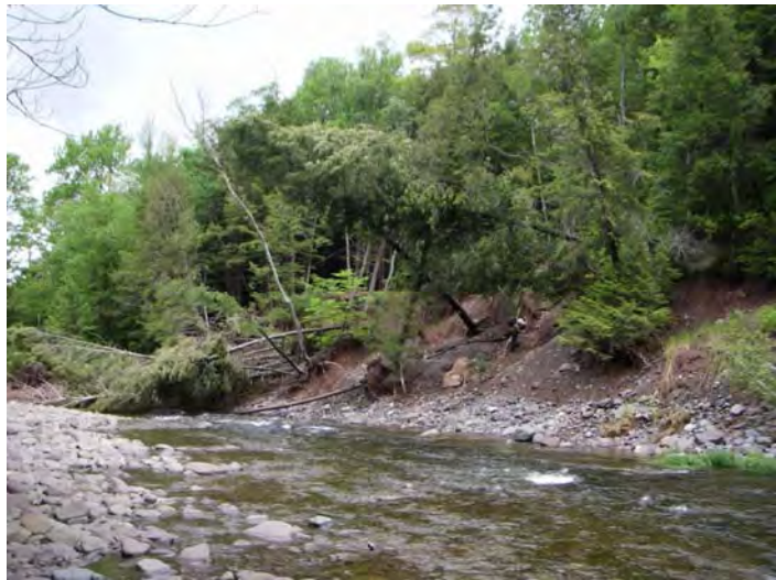
Photo 2.5.5. Hillslope failure in the Schoharie basin
