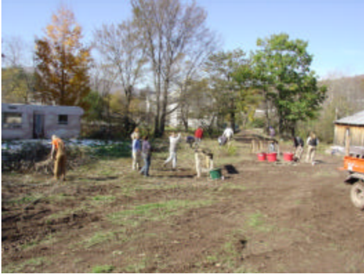
Figure 19: Volunteers tying fascines
