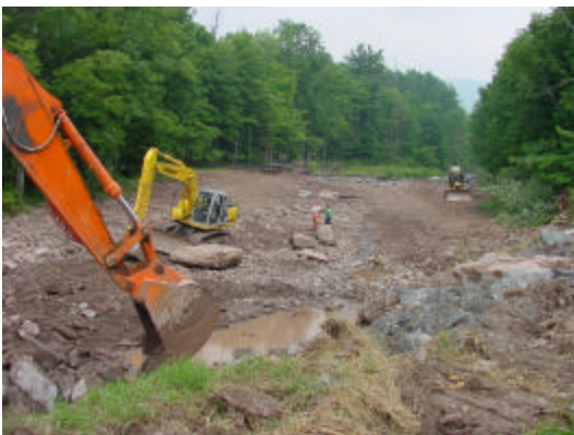
Figure 11: Excavating the design channel
