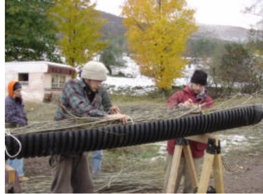
Figure 20: Fascine construction
