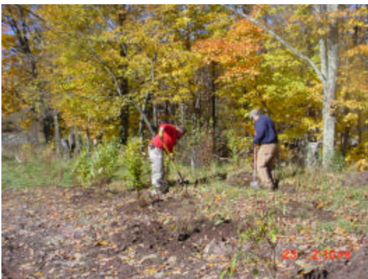
Figure 23: Volunteers installing potted material
