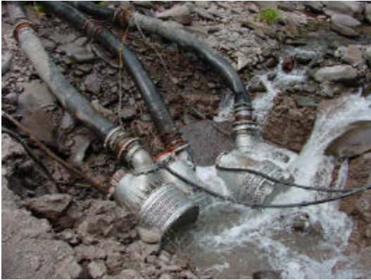
Figure 3: Sump hole for dewatering equipment
