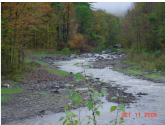
Figure 17: Asbuilt channel after partial bioengineering installation
