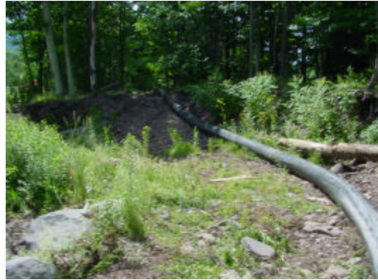
Figure 4: Pipeline used for dewatering
