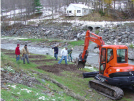
Figure 21: Fascine installation
