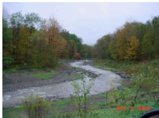
Figure 18: Asbuilt channel after partial bioengineering installation
