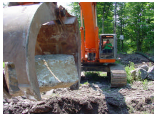
Figure 12: Cross-vane construction
