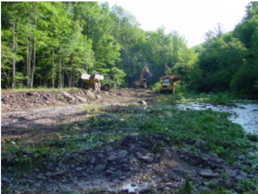
Figure 5: Clearing and grubbing the design channel
