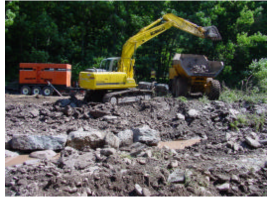
Figure 10: Excavating excess clay from the channel bottom
