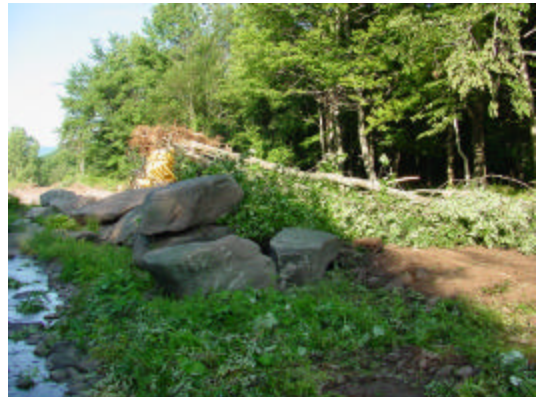
Figure 6: Clearing and grubbing the design channel
