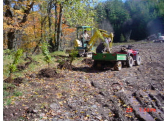
Figure 22: Installation of potted material
