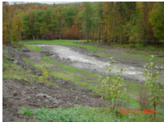
Figure 16: The asbuilt channel after partial bioengineering installation
