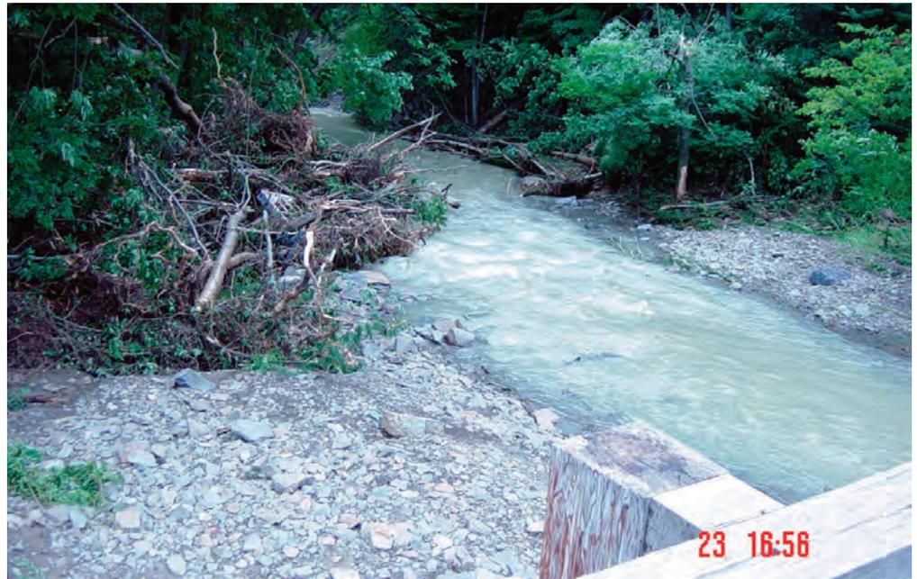
A debris jam caused floodwaters to backup under the bridge and deposit gravel. Partial removal of the debris enabled the stream to re-establish normal flow conditions. *(Photograph courtesy of Melissa Yearick, Upper Susquehanna Coalition.)*
