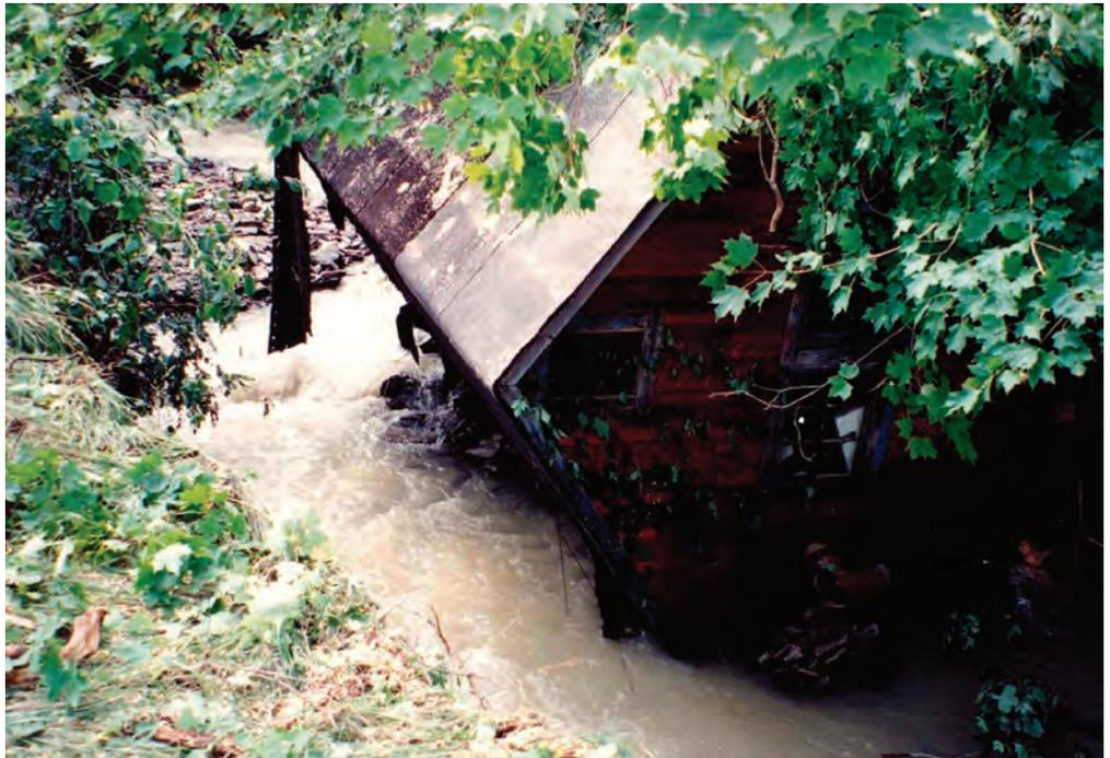
This house was completely undercut by streambank erosion and toppled into the stream. (Photograph by Mark Watts, Chemung County Soil and Water Conservation District.)
