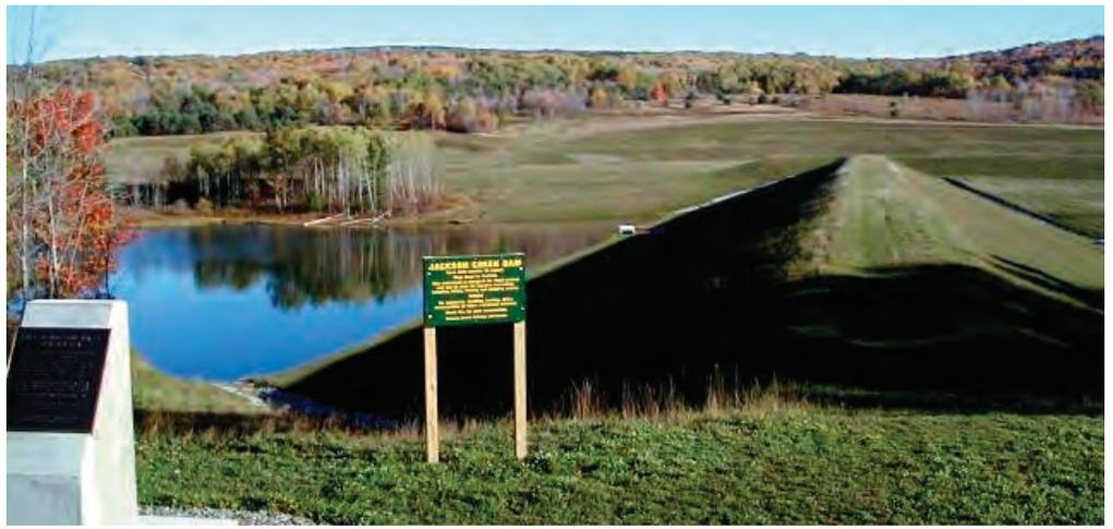
A dam is a barrier or wall constructed across a watercourse or valley to create a reservoir, prevent flooding, capture and store sediment, and/or improve navigability. Dams change the hydrology of a stream by reducing peak flows and providing a steady flow of water for longer periods.
