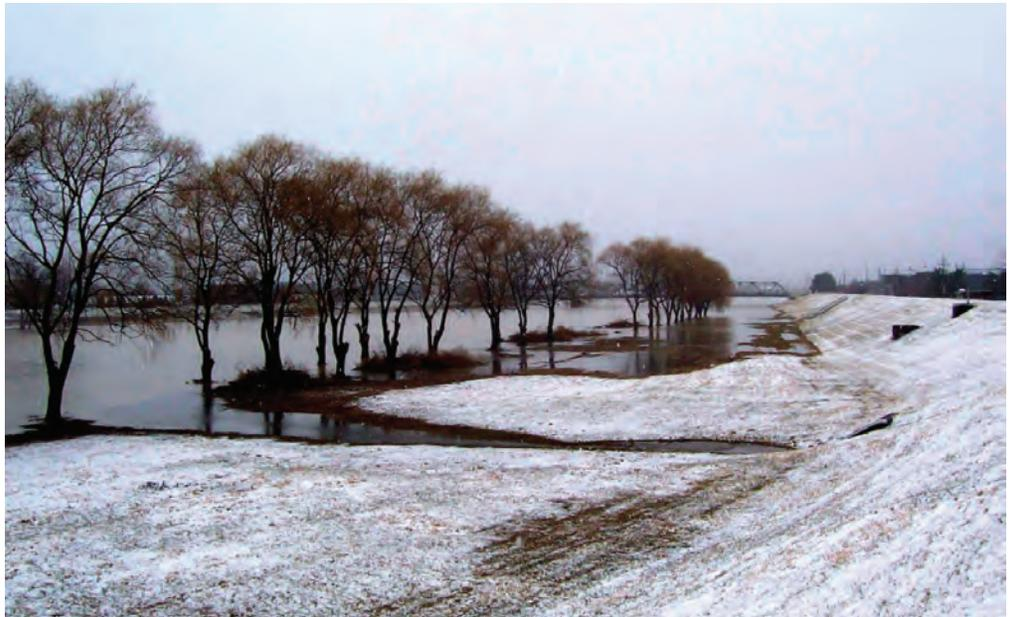
Some flood control dikes are set back from the stream. This allows the stream to function naturally while still protecting nearby land from flooding. Setback dikes maintain a portion of a natural floodplain and provide a floodway where high velocity water can spread out and slow down. *(Photograph by Scott Rodabaugh, NYS Department of Environmental Conservation.)*
