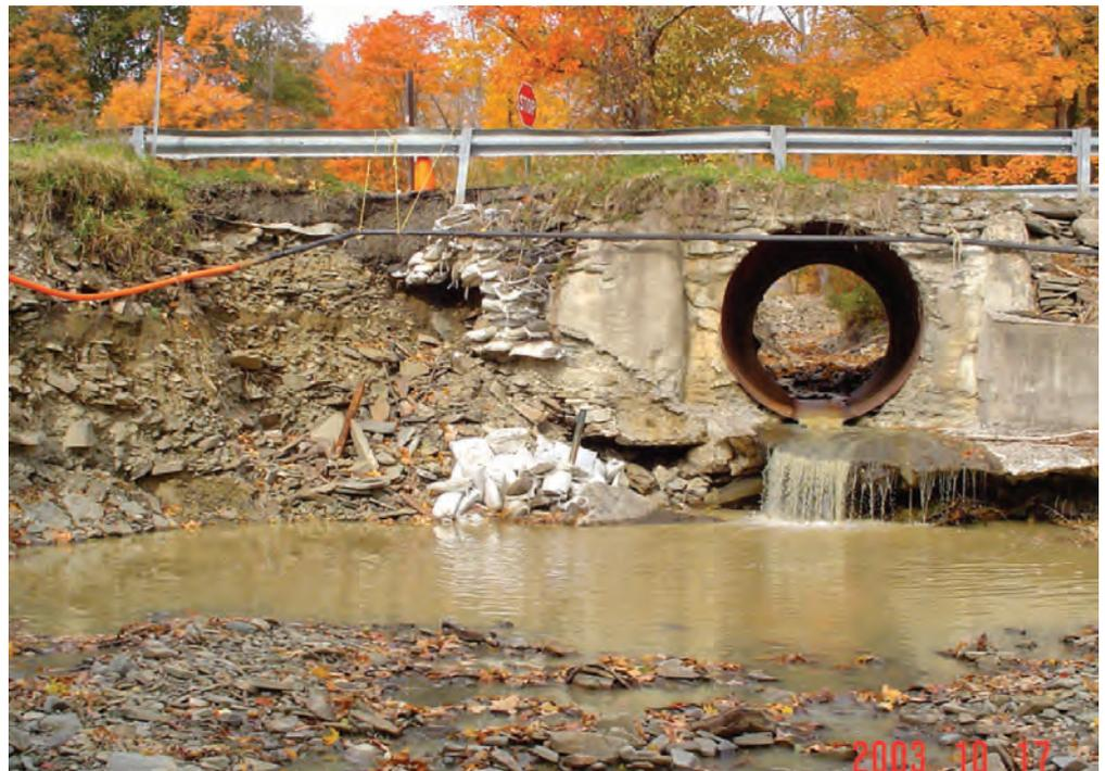
Water shooting out of this culvert has blown out the banks of the downstream channel. *(Photograph by Mark Watts, Chemung County Soil and Water Conservation District.)*
