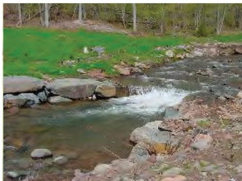
In-stream rock structures can be used to stabilize the bed of a stream. This cross vane consists of large rocks placed in the stream with a "V" shape pointing in the upstream direction. This structure focuses the current toward the center of the channel and away from the banks. Spacing of the boulders enables fish passage and sediment transport through the structure. *(Photograph courtesy of Greene County Soil and Water Conservation District.)*
