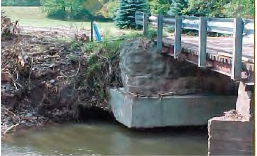
This scour under a bridge is a good visual indication of stream down cutting or degradation. *(Photograph courtesy of Greene County Soil and Water Conservation District.)*
