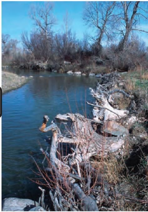
Trees have been buried and anchored in the streambank so that the root wads provide erosion protection. (Photograph by Gary Kramer, USDA Natural Resources Conservation Service.)
