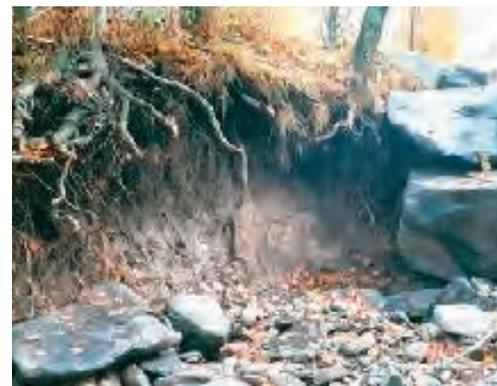
Streambank erosion can occur adjacent to or even behind rock riprap. (Photographs courtesy of Greene County Soil and Water Conservation District.)
