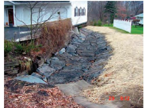
This house was constructed so that a portion of the structure extended over the stream. The builder apparently did not anticipate that the stream would erode its channel ten feet deep and undermine the building foundation (left photo). In order to protect the house, the creek bed was raised, lined with rock, and stabilized with a drop structure – at a cost of \$36,000 (right photo). (Photographs by Gary M. Patelunas, Town of Elmira Stormwater Department.)
