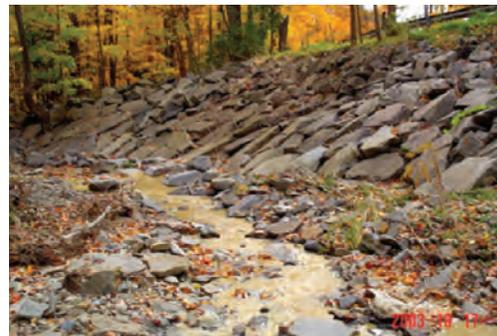
Rock riprap is probably the most familiar of all streambank protection methods and can be an effective means of protecting streamside development. (Photographs by Mark Watts, Chemung County Soil and Water Conservation District.)
