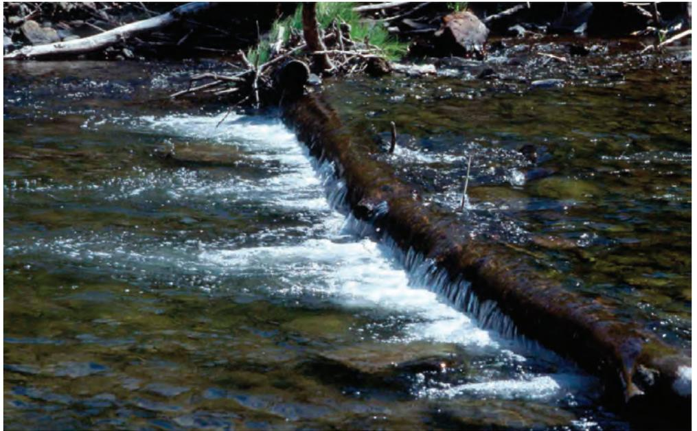
Fallen trees or anchored log structures function in much the same way as check dams for channel gradient stabilization. *(Photograph by Gary Wilson, USDA Natural Resources Conservation Service.)*
