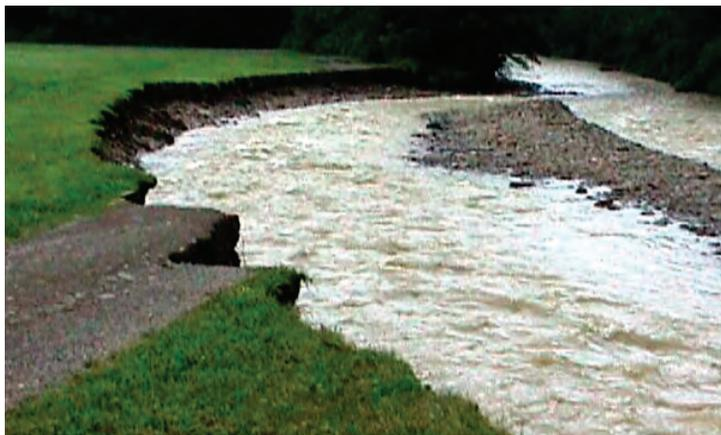
Flooding of this stream caused a washout extending 100 feet into the adjacent field. The site was restored by filling in the washed out area, stabilizing the bank with rock riprap, construction of two in-stream rock structures, and planting willows along the edge of the field. *(Photographs courtesy of Steuben County Soil and Water Conservation District.)*
