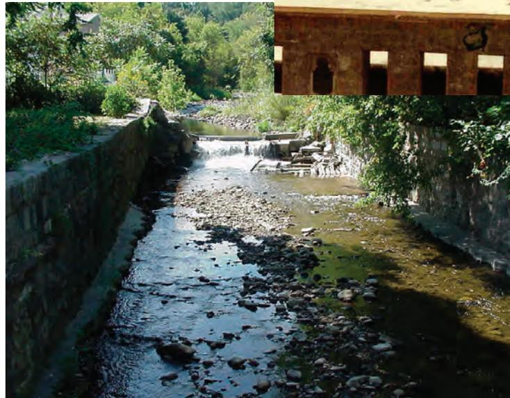
This channel was designed to carry a stream safely through a residential neighborhood. Unfortunately, the narrow channel and a low bridge clearance restrict the flow of ice, causing ice jams at this location. (Photographs courtesy of Herkimer-Oneida Counties Comprehensive Planning Program.)
