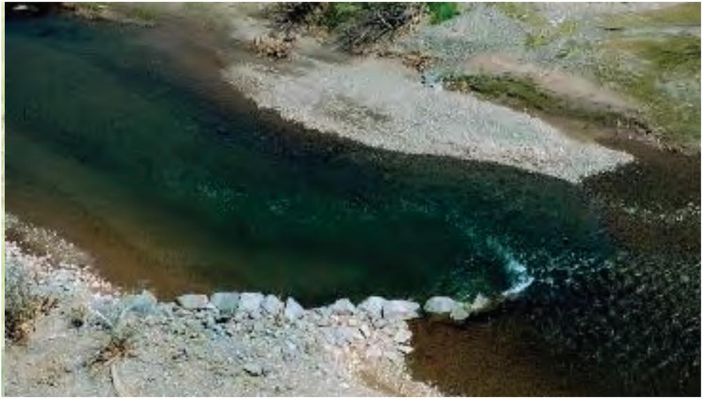
Rock vanes are carefully placed rock structures built below the water level to control the direction of flow within a stream. This vane reduced the velocity adjacent to the streambank, resulting in sediment deposition near the bank on the upstream side of the structure. Vegetation can be planted on this newly deposited material to provide additional protection. *(Photograph courtesy of Greene County Soil and Water Conservation District.)*
