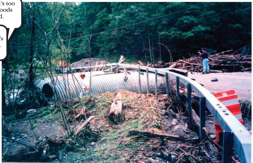
The design of some bridges and culverts is simply not large enough to allow for the high flow and debris associated with a major flood event. When fast moving floodwater is funneled through an undersized structure, the bridge or culvert may be overtopped, damaged by erosion, or even washed out. (Photograph courtesy of Herkimer-Oneida Counties Comprehensive Planning Program.)
