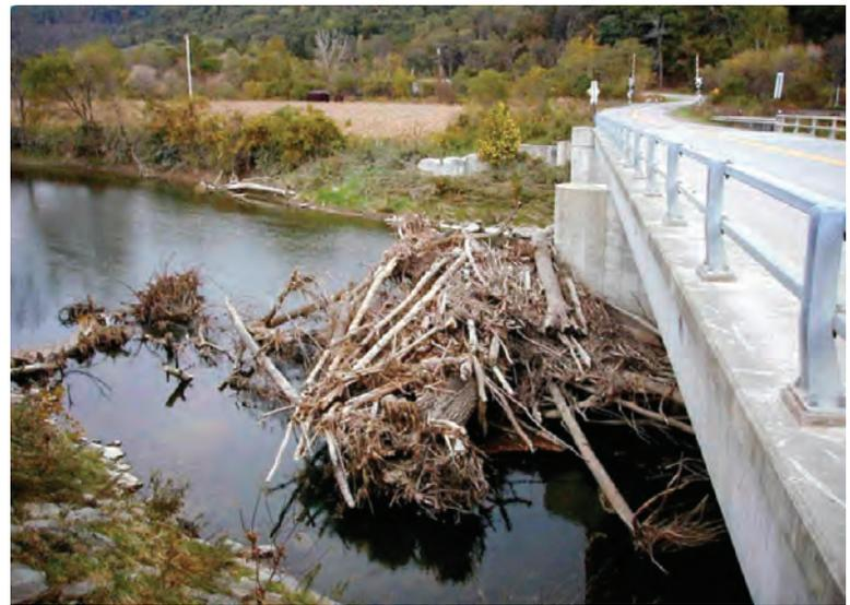
Debris can threaten any bridge or culvert, but if a bridge pier or multiple culvert design splits the stream flow, the risk of debris damage is increased. *(Photographs by Gary M. Patelnas, Town of Elmira Stormwater Department and Scott Rodabaugh, NYS Department of Environmental Conservation.)*
