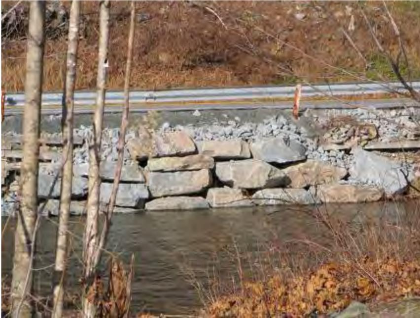
**Figure 8:** *Large Rocks Protecting and Stabilizing Stream Bank Adjacent to Road Infrastructure* (New York City DEP, 2008b).
