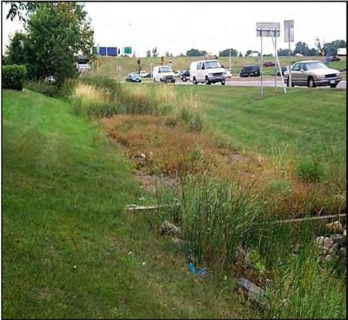
**Figure 72:** *Highway Right of Way Vegetative Swale* (Schueler et al., 2007).
