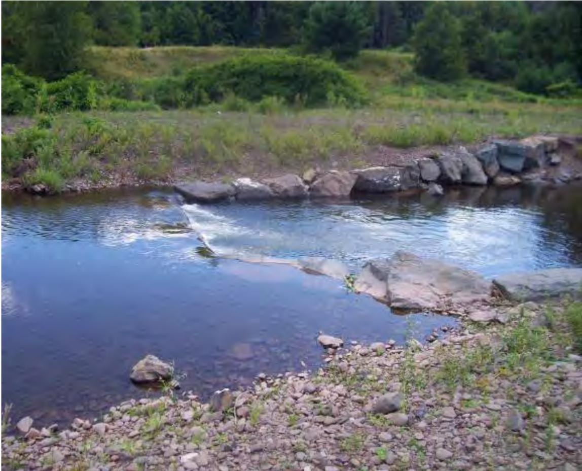
**Figure 64:** *Cross Vane Rock Structure, Greene County, NY.*
