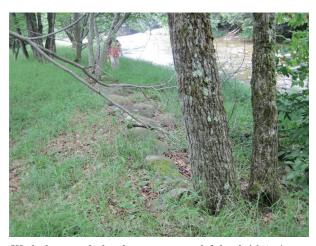
Washed out stacked rock revetment on left bank (A174)
