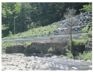
Stacked rock revetment on concrete and bedrock foundation (A302)
