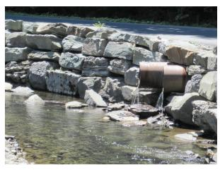
Stacked rock revetment protecting Frost Valley Road (A282)
