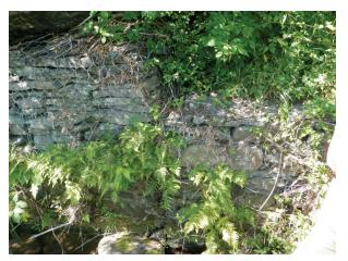
Stone gabion revetment on right bank (P7190130)
