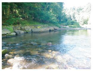
Placed quarry rock forming grade control (P7290125)
