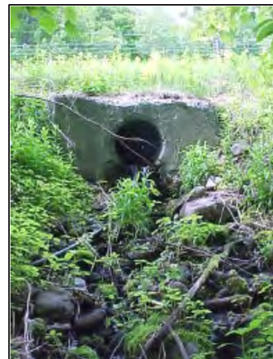
Figure 12 Culvert outfall
