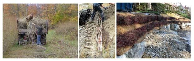
Live dormant willow cuttings are often used to make stakes and fascines, as seen in the first two photographs above. The last photograph shows how vegetation can be incorporated into a traditional bank armoring project to provide habitat, cooler water temperatures through shading and long-term stability for the project.
