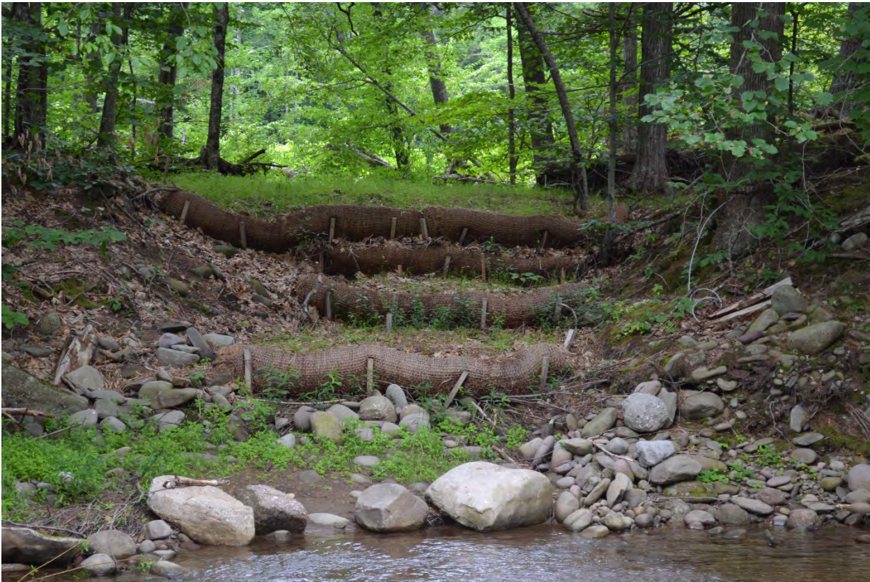
BIOENGINEERING AT CLARYVILLE ABOVE CONFLUENCE OF E. AND W. BRANCH NEVERSINK 2017
