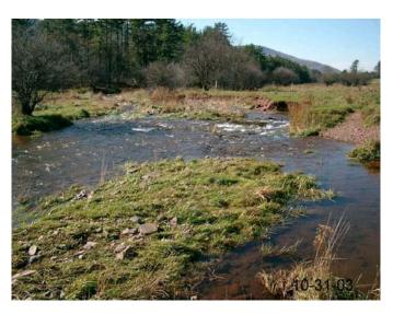
A 1500 ft. headwater reach of *Town Brook in the Town of Stamford on the David Post farm* was restored using natural channel design methods and structures in 2004. Bank erosion and stream bed degradation along this reach was introducing phosphorus laden agricultural soils into waters where phosphorus was a target of water quality improvement efforts (see photo at left)
