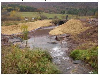
medium rock riprap interplanted with live cuttings of willow and the construction of a cross vane to direct flows and prevent headcutting upstream. The project protects areas planted as a riparian buffer under the CREP.
