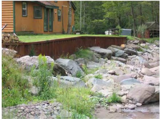
**Figure 7:** *Steel Sheet Pile Wall Protecting Private Property From Stream* (New York City DEP, 2008b).
