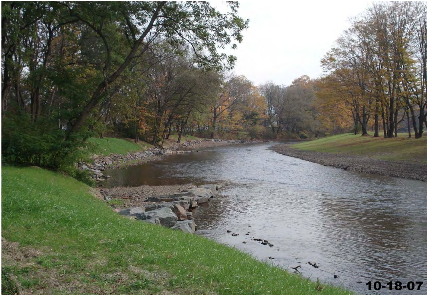
Margaretville Pavilion Park Streambank Stabilization - 2007
