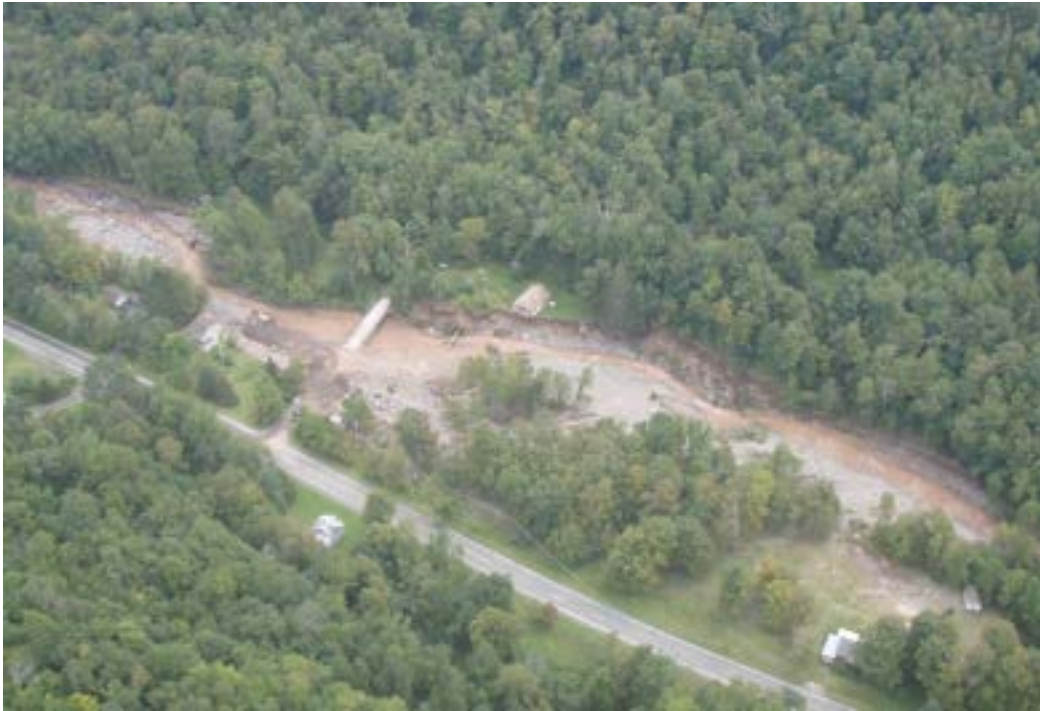
Photo 3-8 Erosion damage at the Wright Road bridge during Tropical Storm Irene in 2011. Repairs to approach roadway embankment are underway. Photo provided by NYCDEP SMP.
