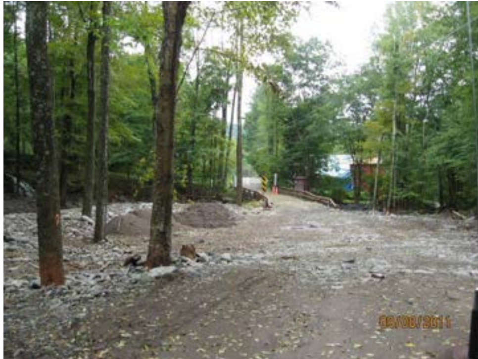
Photo 3-12 Diamond Notch Road bridge over Hollow Tree Brook following 2011 flooding. Note damage to roadway from overtopping. Photo provided by HLFRC.
