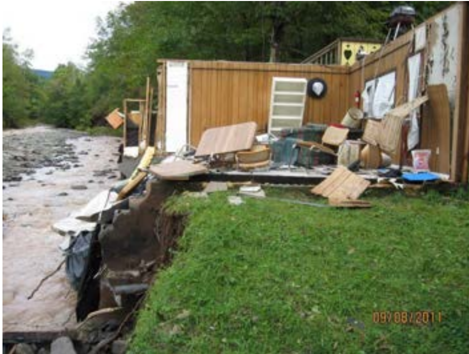
Photo 3-19 Home alongside Stony Clove Creek in Meadow Brook Drive neighborhood (Section 3.1.2) destroyed by stream bank erosion in 2011. This home went through the FEMA buyout process and the parcel is now owned by the NYCDEP. Photo provided by HLFRC.
