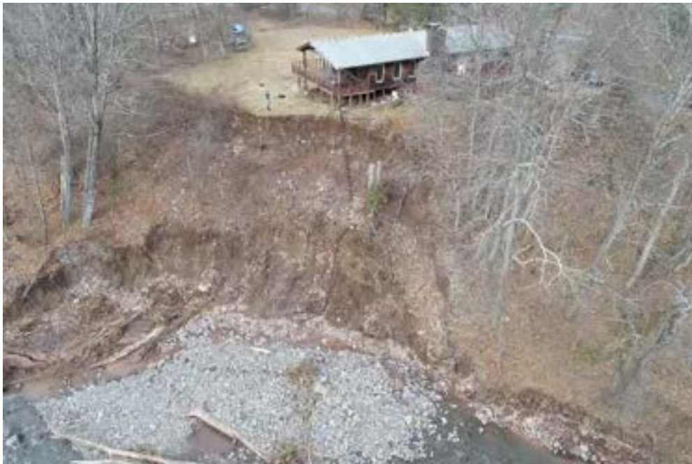
Photo 3-18 Stream bank-coupled hillslope failure along a dynamic reach of Stony Clove Creek (see Figure 3-35) threatening adjacent structure. January 1, 2021, photo. This property was purchased through the NYCFFBO due to erosion hazard risk.
