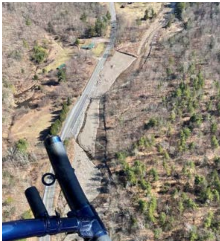
Photo 3-4 Repairs to NY-214 following damage in December 2020. Stony Clove Creek was relocated farther from the road. Photo provided by NYCDEP SMP.
