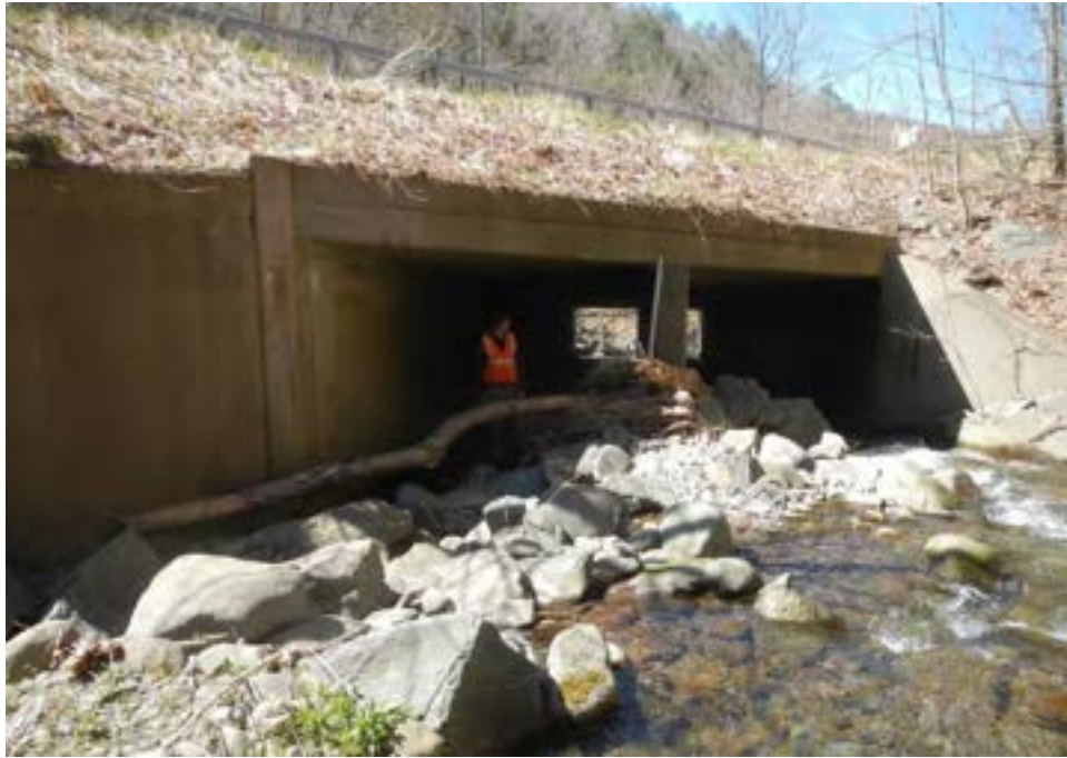
Photo 3-13 NY-214 culvert over Myrtle Brook – inlet, looking downstream. Note partial obstruction by wood and sediment.
