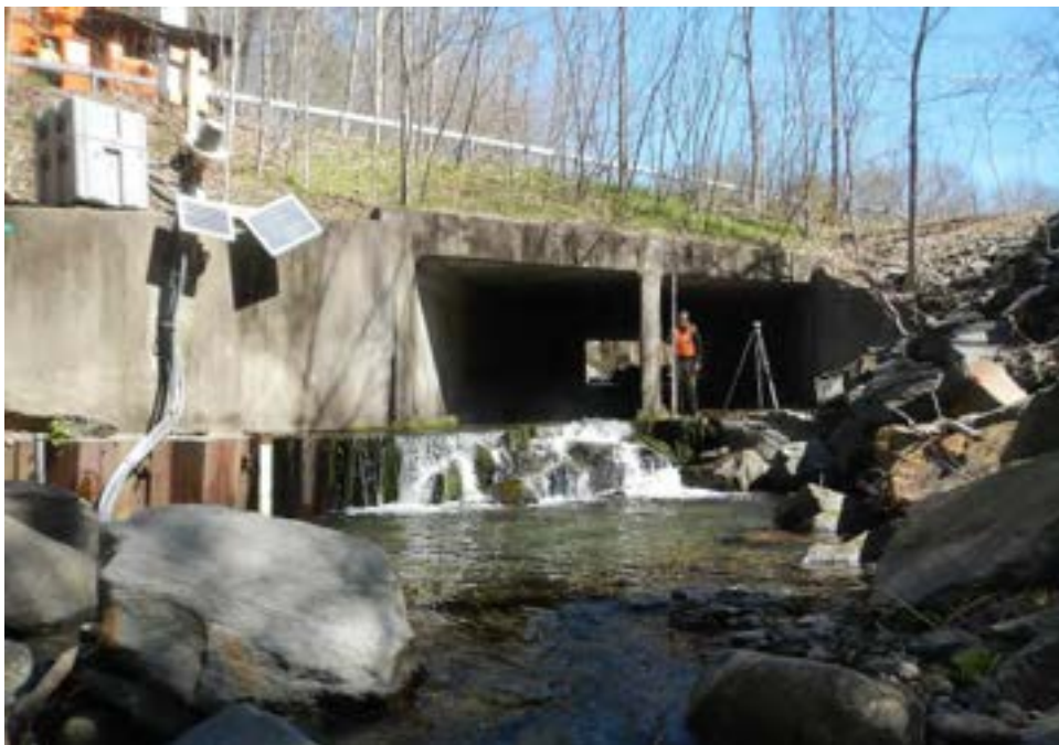
Photo 3-14 NY-214 culvert over Myrtle Brook – outlet, looking upstream. USGS gauging station at left. Note sheet piling and aquatic organism barrier.
