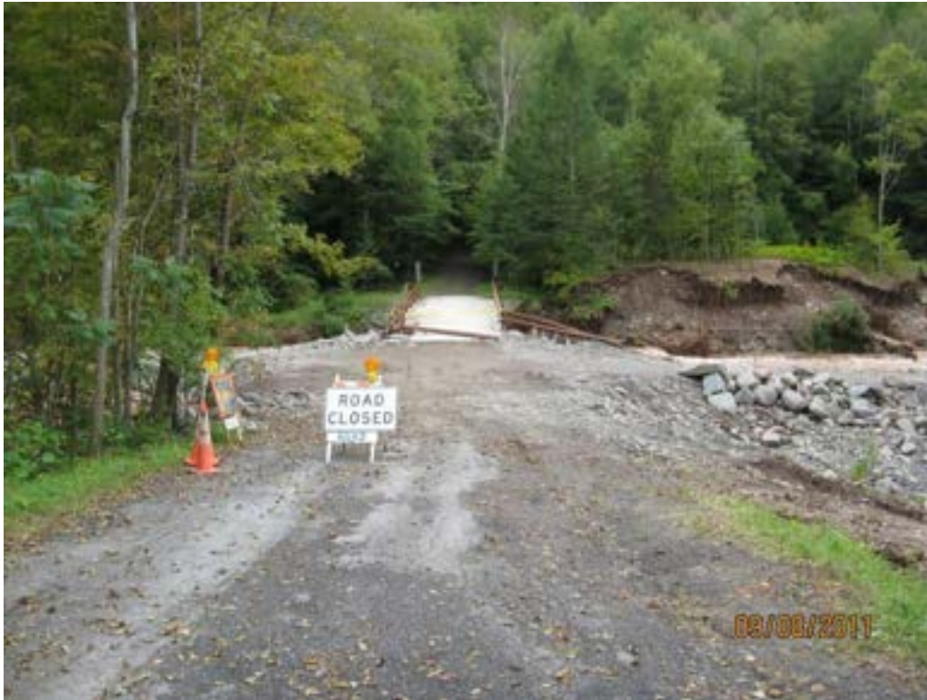
Photo 3-9 Damage to Wright Road bridge in 2011 flooding. Photo provided by HLFRC.
