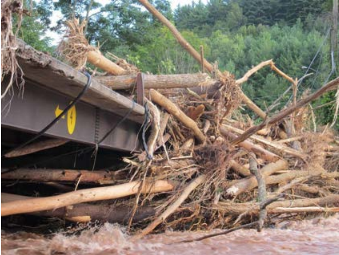
Photo 3-23 Large wood accumulation at Bridge Street bridge over Esopus Creek in Phoenicia during Tropical Storm Irene in 2011. Photo provided by Amy's Takeaway.
