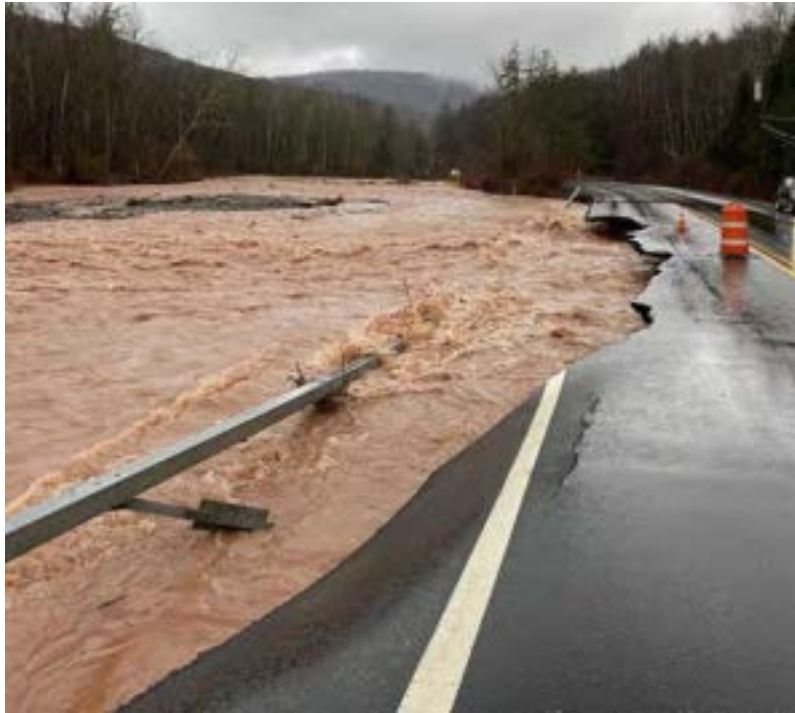
Photo 3-1 December 2020 flood damage to NY-214. Photo provided by AWSMP.
