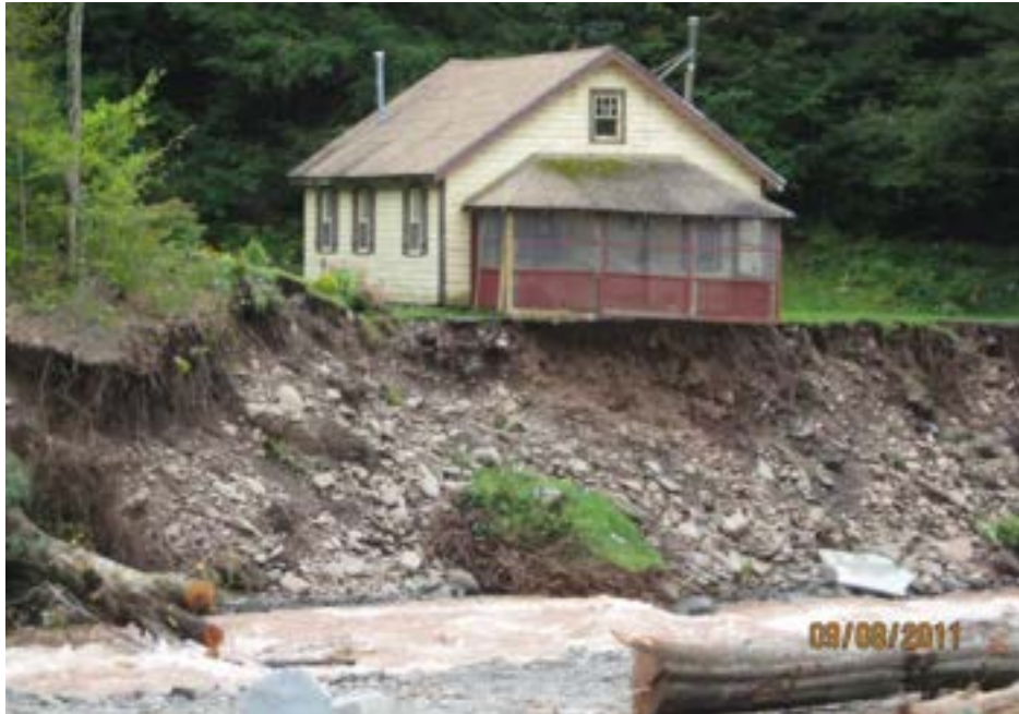
Photo 3-17 Damage to home along Stony Clove Creek from bank erosion in 2011 flooding. Photo provided by HLFRC.
