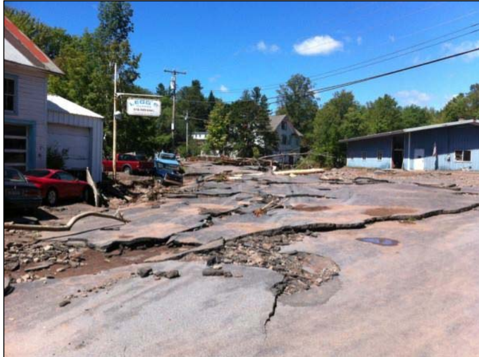
Figure 9. Tannersville properties immediately following Tropical Storm Irene. The Highway Garage is on the right and the property condemned by Greene County is in the center background.
