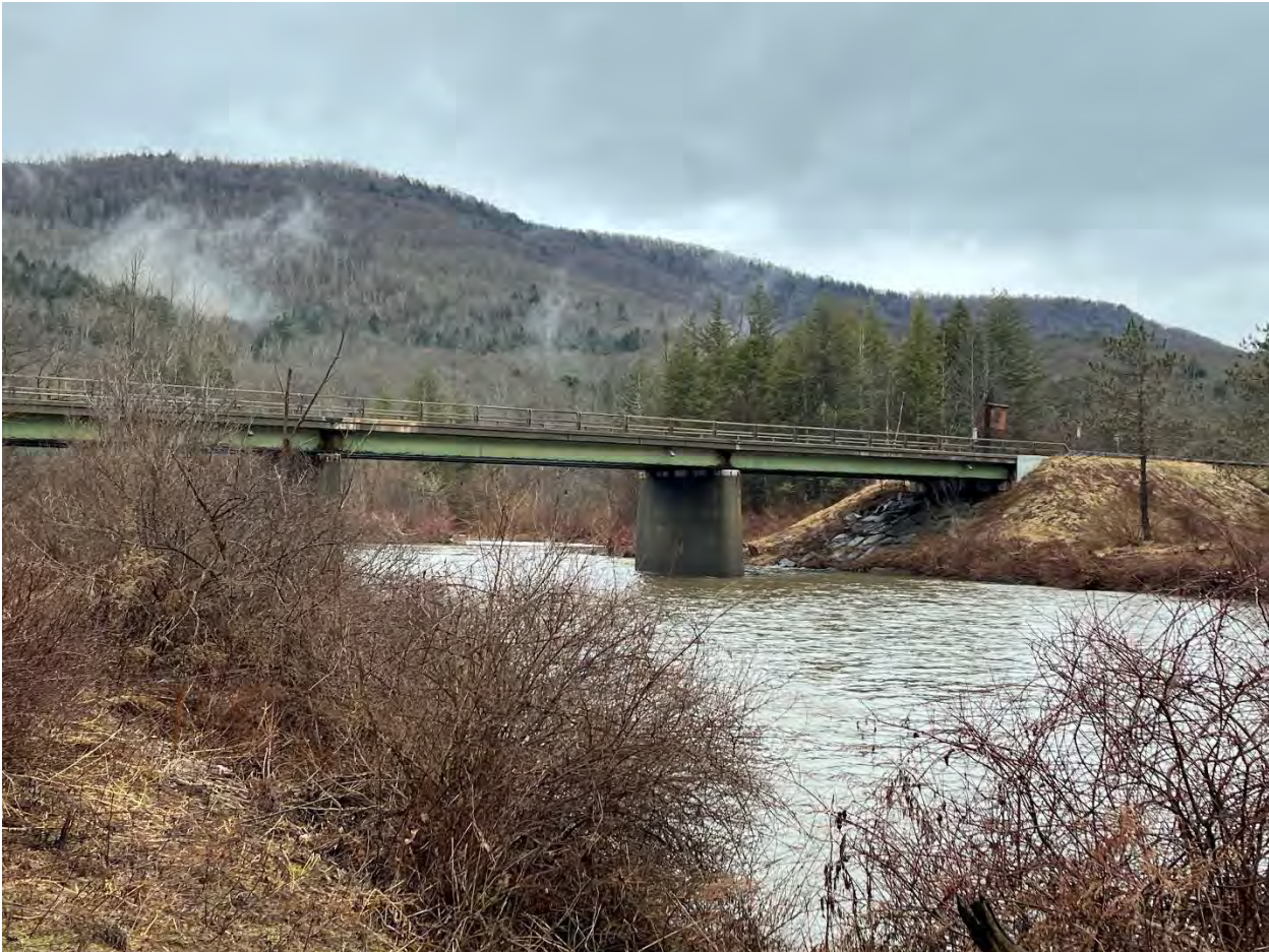
Figure 4-26: Route 28/30 bridge over the EBDR
