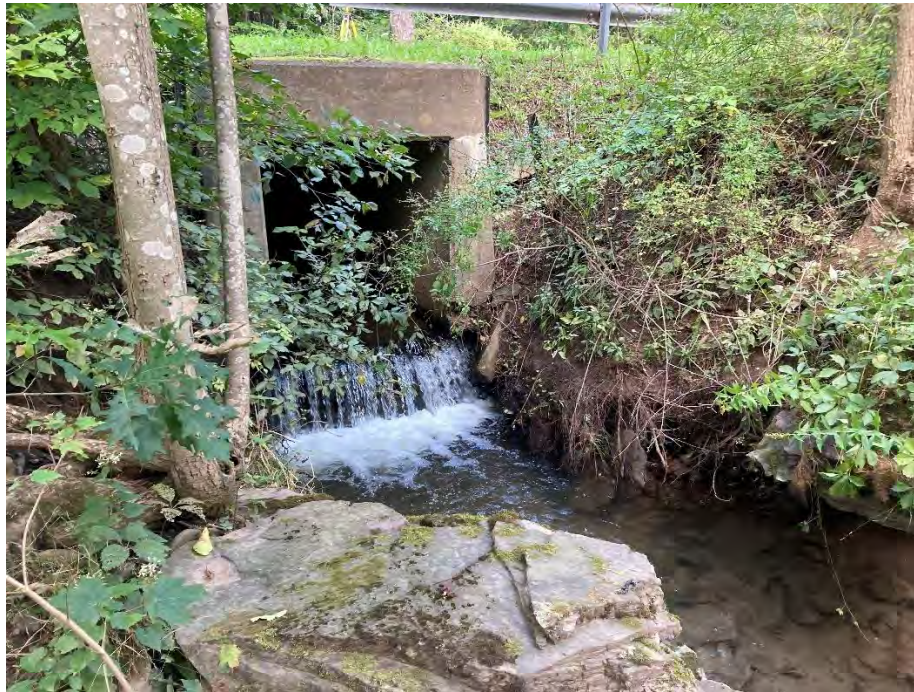
Figure 4-25: Outlet of Scott's Brook culvert under Main Street
