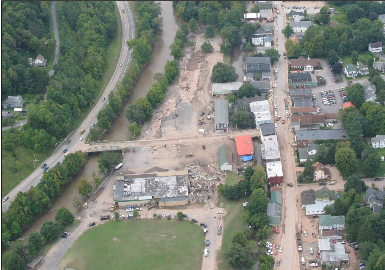
Figure 4-6: Damage in Margaretville, near Bridge Street, after Tropical Storm Irene (Photo courtesy of NYCDEP Stream Management Program)
