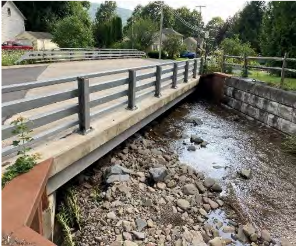
Figure 4-18: Inlet of Swart Street bridge over Bull Run with low-flow channel
