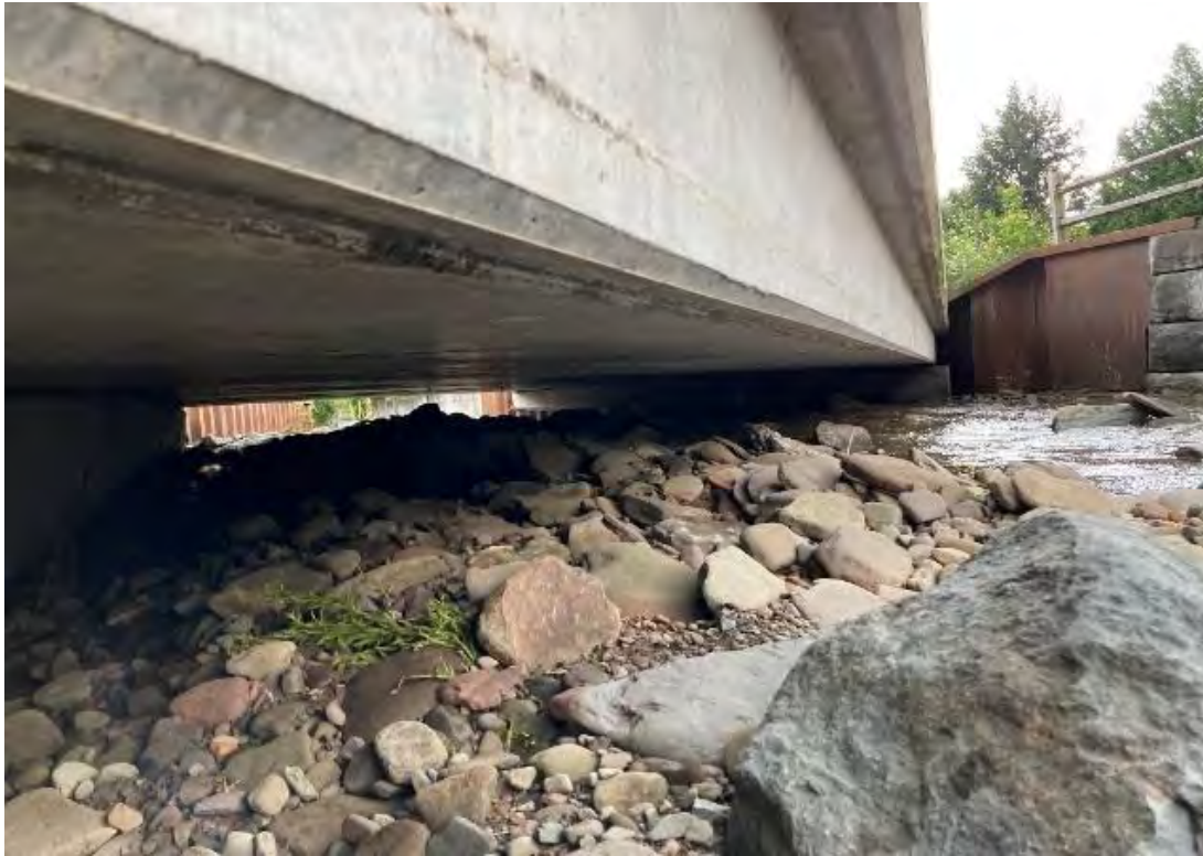
Figure 4-19: Sediment has deposited under the Swart Street bridge, reducing the rise to about 2 feet on the northeast side
