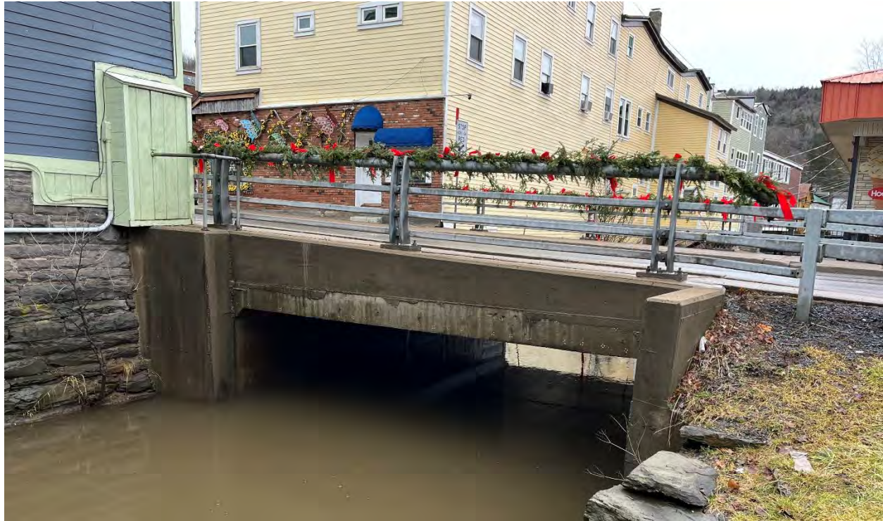
Figure 4-7: Bridge Street bridge over the Binnekill (BIN 1020840)
