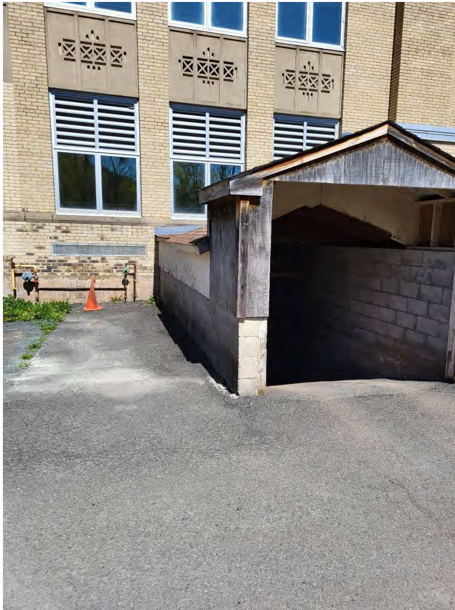
Figure 4-29: Ramp access to basement of Margaretville Central School
