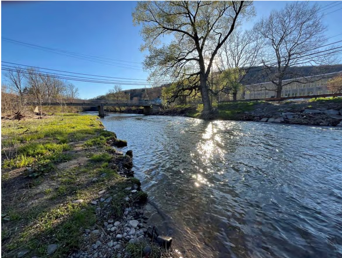
Figure 4-12: Sediment bar on upstream side of Fair Street bridge
